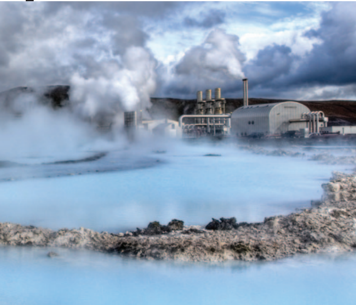
Left: Svartsengi power plant in Iceland.
